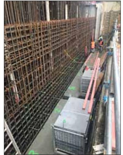
Two new 10-storey shear walls to secure the Bowen State Building required 130 tonnes of reinforcing and 380m<sup>3</sup> of concrete.
