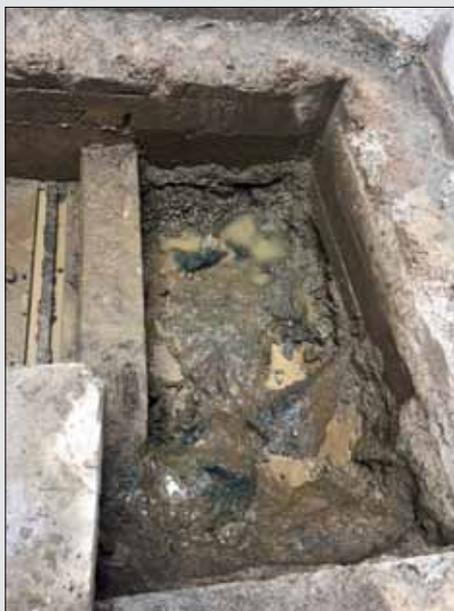
◀ PHOTO: The volcanic lava flow beneath the building. It lies directly under the existing footings which had been cut into it. Across the wider Auckland area, there are 48 volcanic cones.
